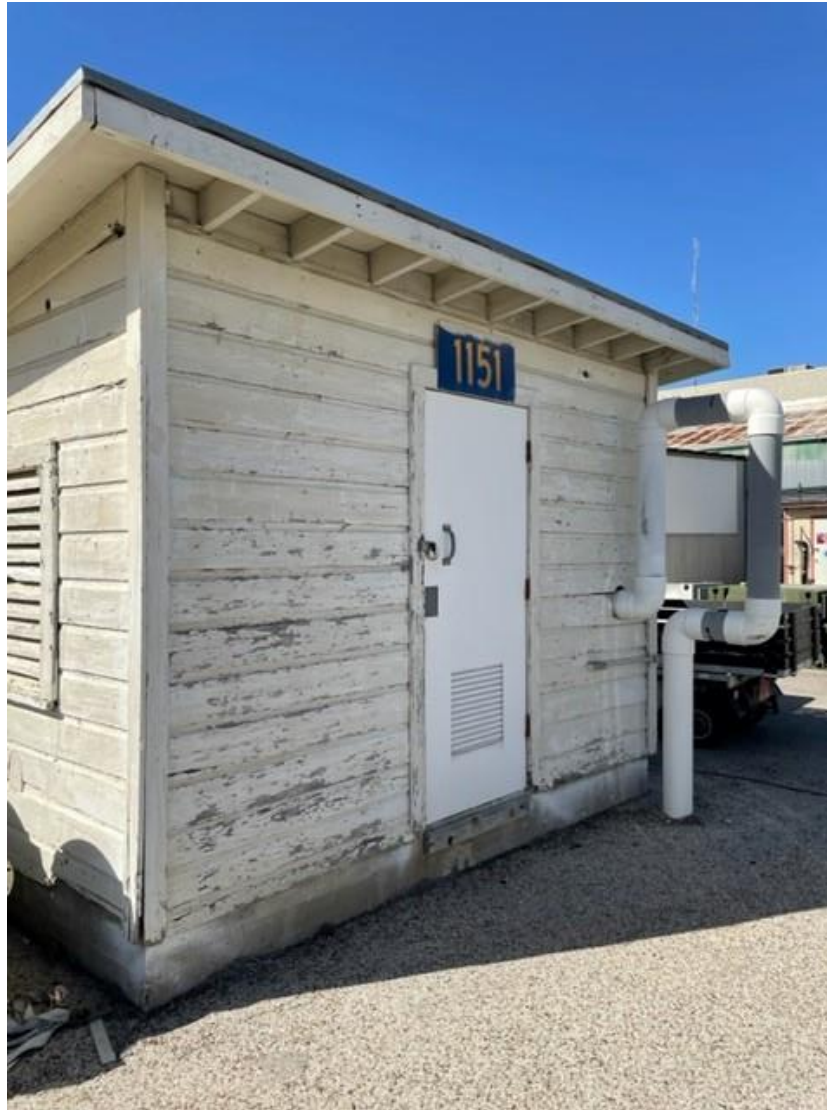
Lift Station 1151 was built in 1944. Its capacity is one million gallons per day (1 MGD).
