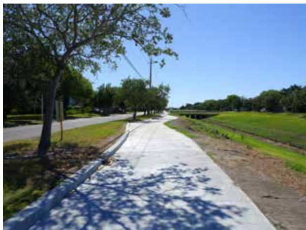
Example of Drainage Facilities Used for Trail Connection - Schanen Hike/Bike Trail
