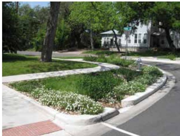
Example of Bioswale Drainage
