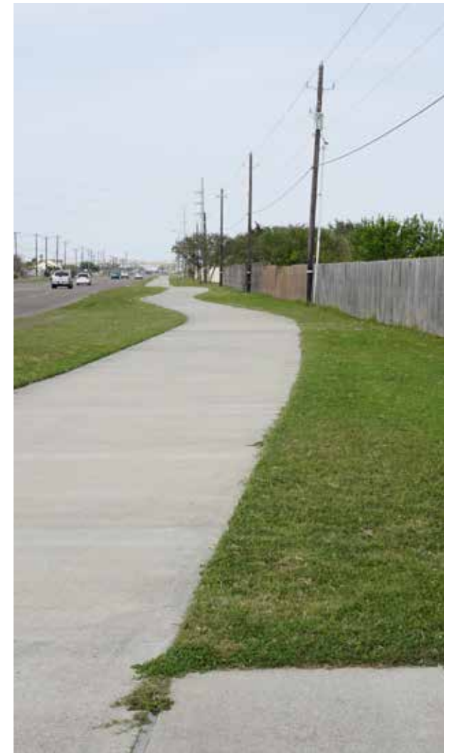
Existing Sidewalk along Flour Bluff Drive
