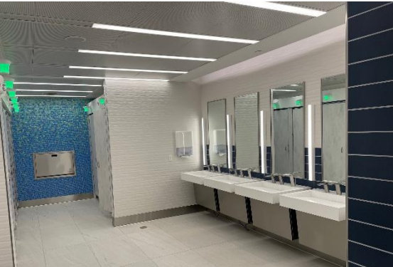
New fixtures, floor, walls, and ceiling
