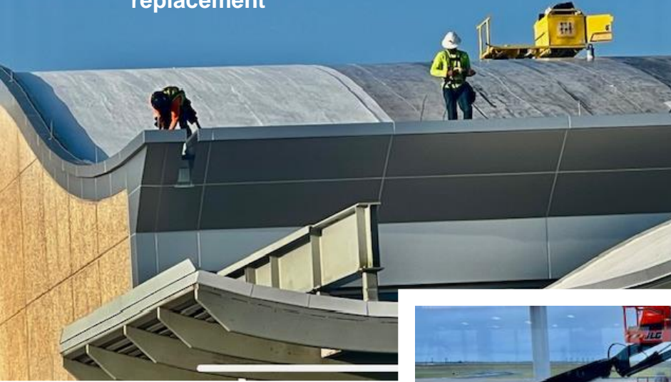
Terminal roof and PVC replacement
