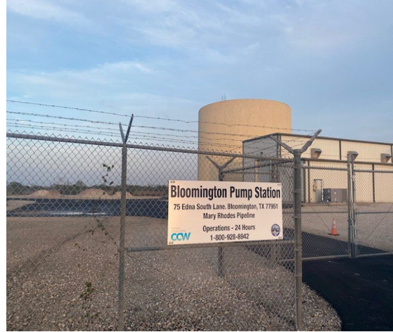
Bloomington Pump Station
