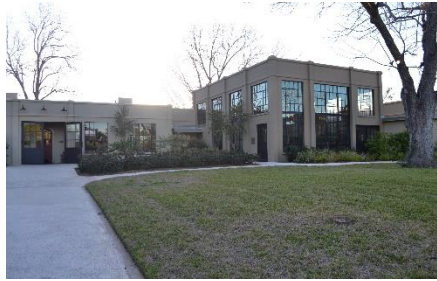
Pump House Victoria, TX
