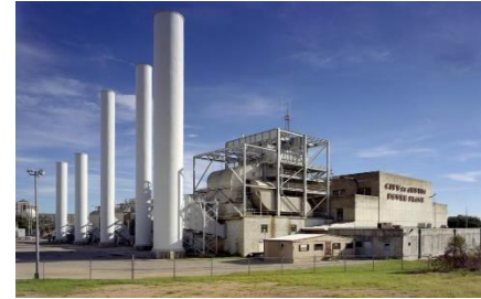
Boiler 9 Austin, TX
