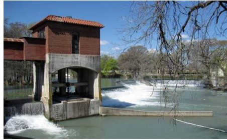
Power Plant Texas Grill Seguin, TX
