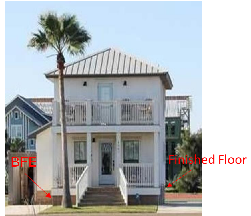
Pier and Beam
