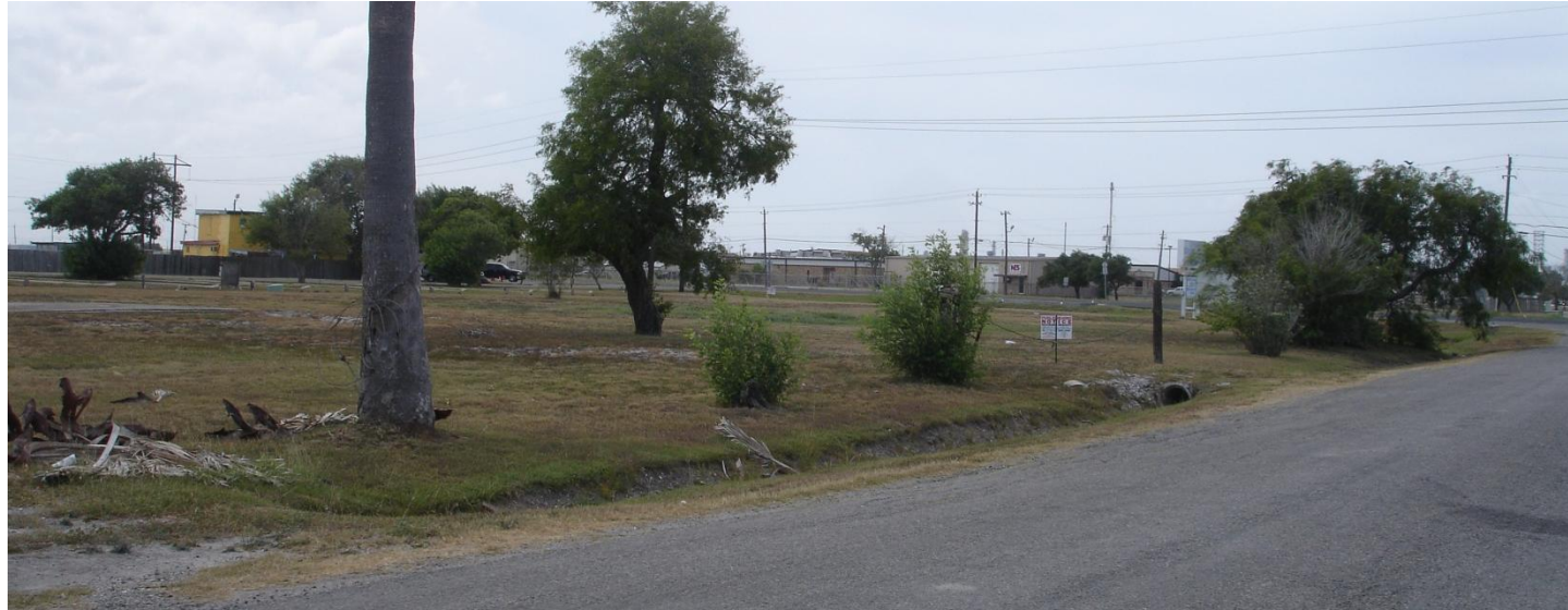
Northwest Along Stillwell Lane toward Tuloso Road
