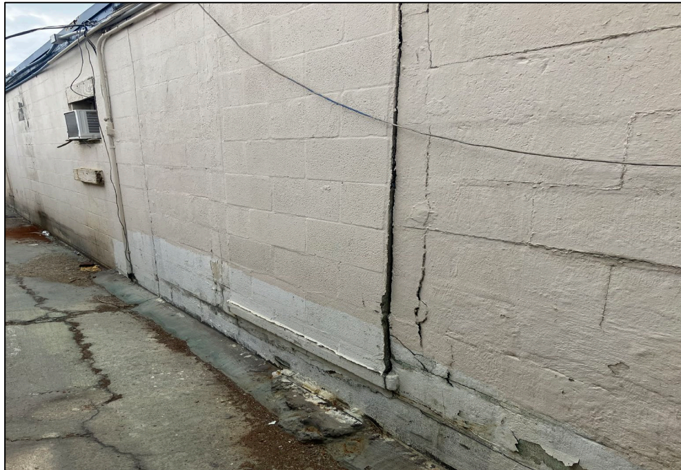
Northside wall failure and interior water damage
