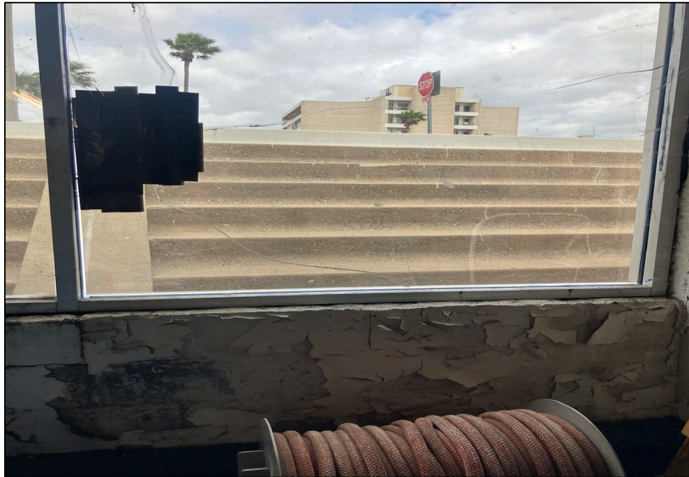
Broken window and rainwater buildup
