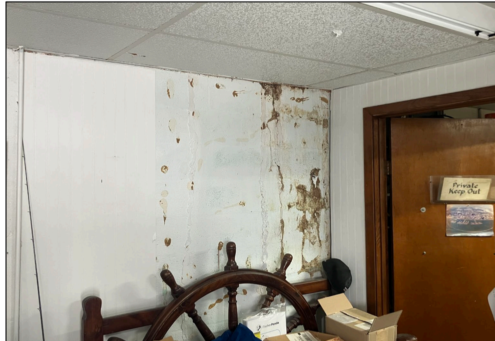
Northside wall failure and interior water damage
