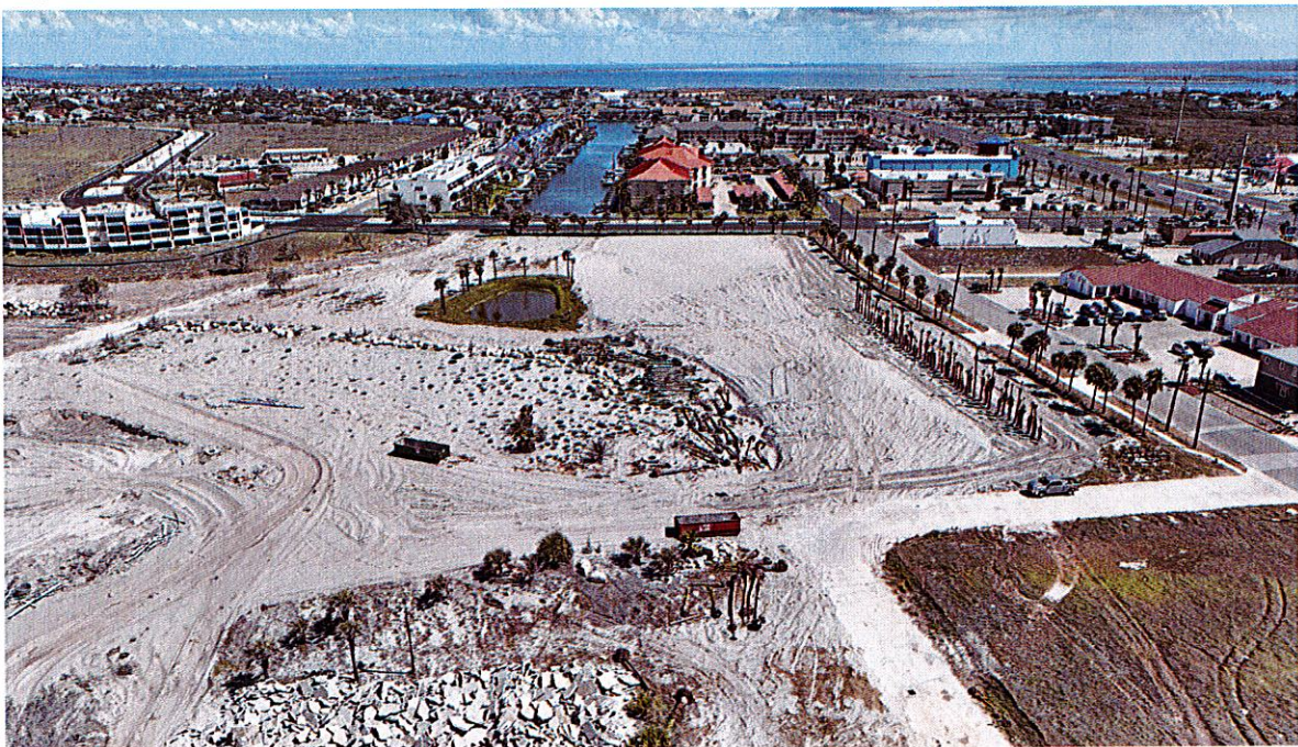
Figure K: Drone Photo of Baseline
