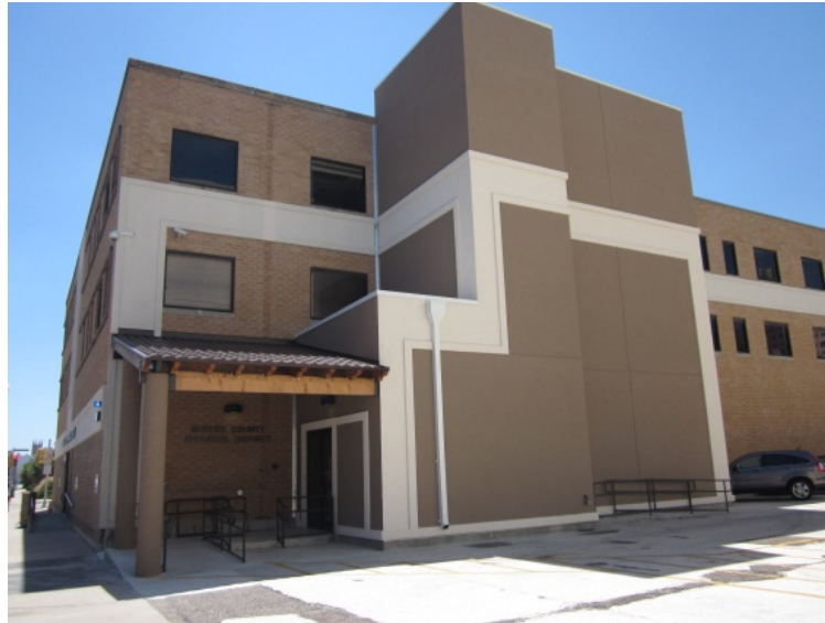
NEW BUILDING ADDITION AND ELEVATOR
