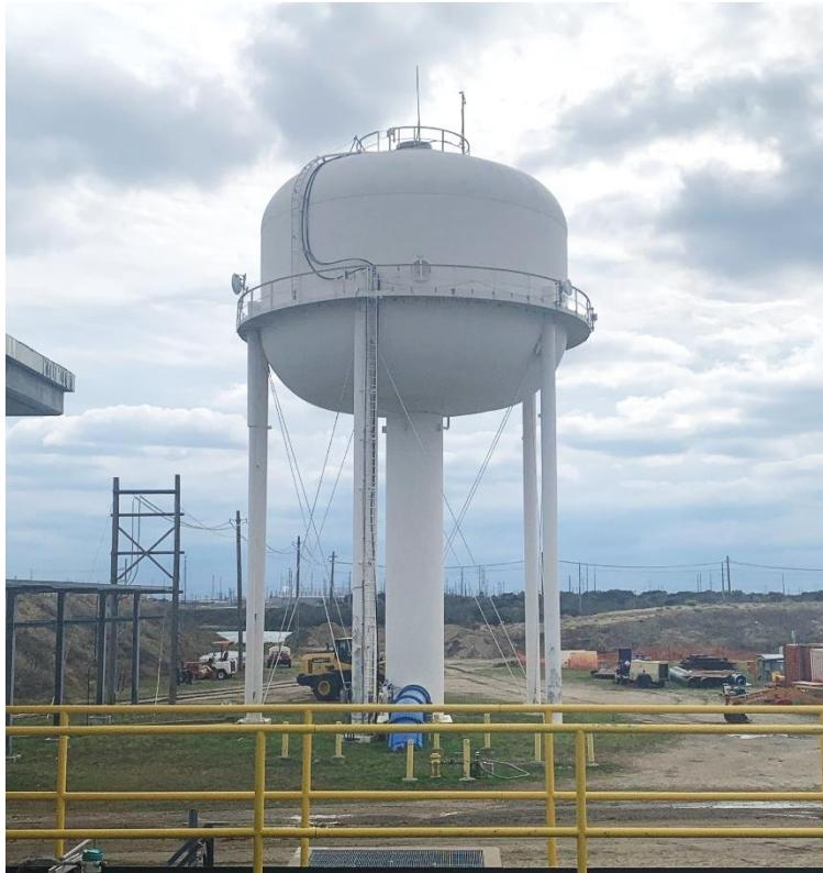
The project scope of work includes the critical restoration and rehabilitation of the ONSWTP Filter Media Backwash elevated storage tank. The Filter Media Backwash tank is critical to maintaining filter effectiveness and overall water quality.
