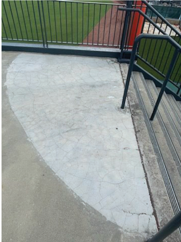
Miscellaneous concrete repairs throughout stadium to eliminate failures and trip hazards
