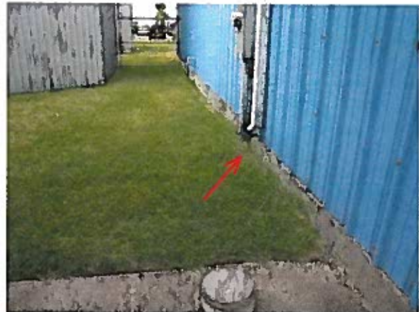
Downspout @ Signature Offices
