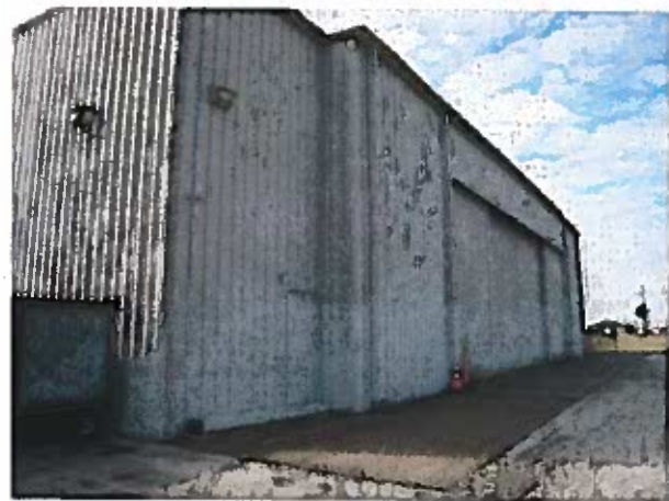
East GA Hangar 3 – Air Side (North)
