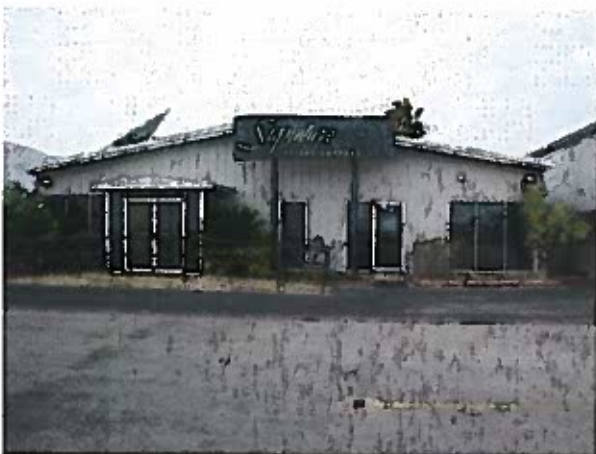
Signature Office Building – Air Side
