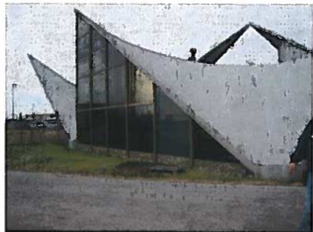
East GA Hangar 1 – SWA Office Area
