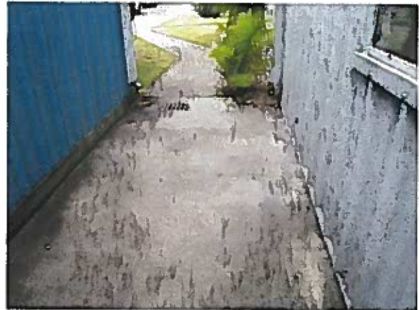
Drain in Good Condition @ OAC
