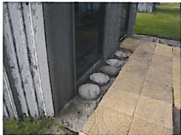
Steps added due to poor drainage
