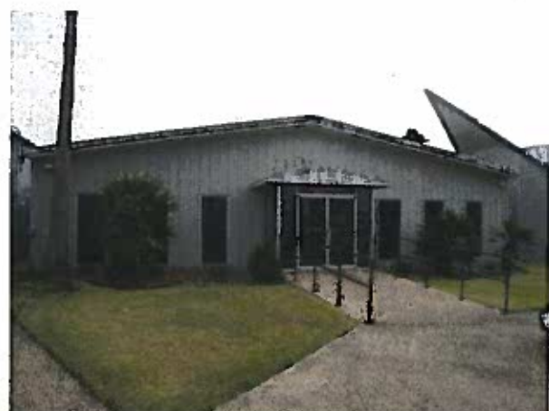
Signature Office Building – Land Side
