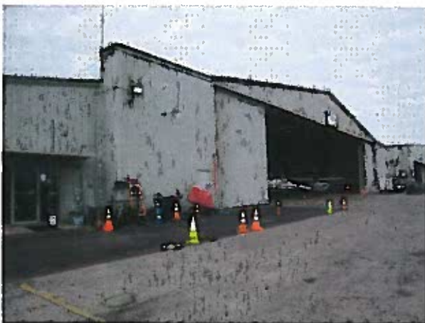
East GA Hangar 2 – Ocean Air Center – Air Side
