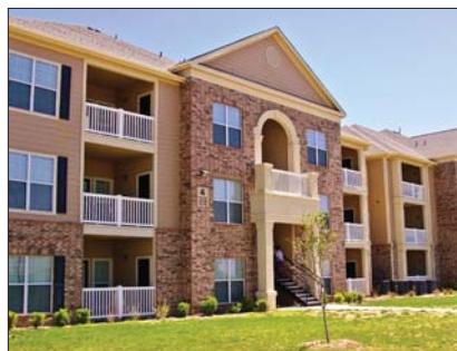
TownParc at Amarillo Apartments in Amarillo.
