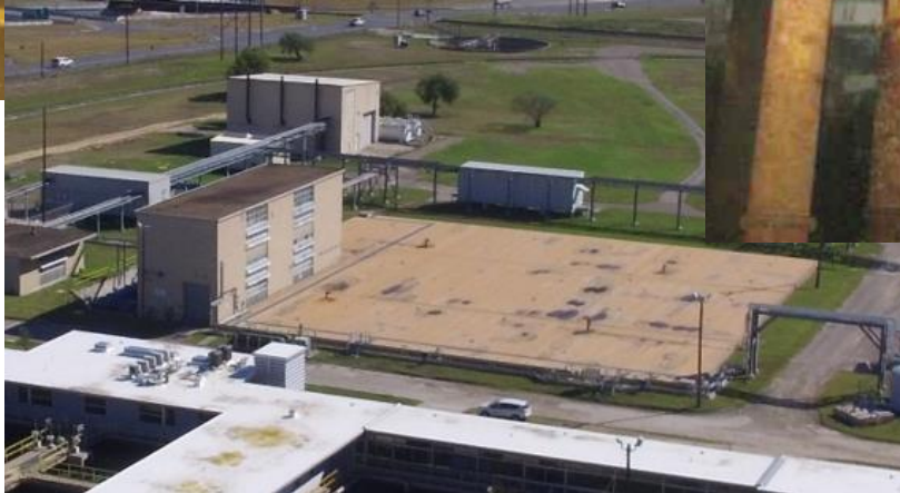
Aerial view of existing Clearwell and pump station →
