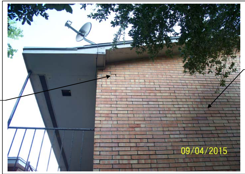
Photograph No. 5 – Typical Cracking Seen in Brick Veneer
