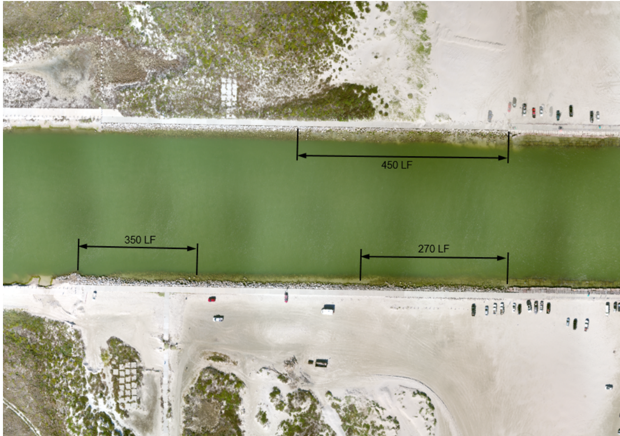
Figure 15 – Landside Jetty Damage Areas in Reach 2.
