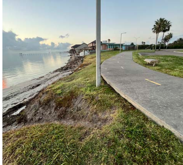
Shoreline erosion at Poenisch Park on the Corpus Christi Bay.
