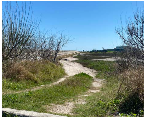
Preventing vehicular access to the Oso Bay shoreline is critical to protect the Bay's natural features from vehicle impacts such as the ground wear pictured above
