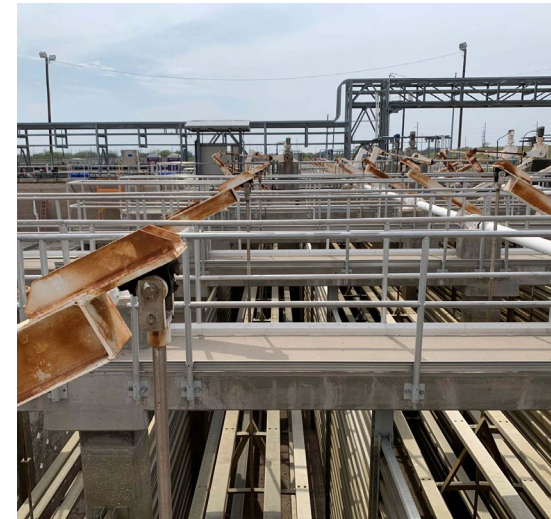
Walking beam flocculator rotating arm corrosion
