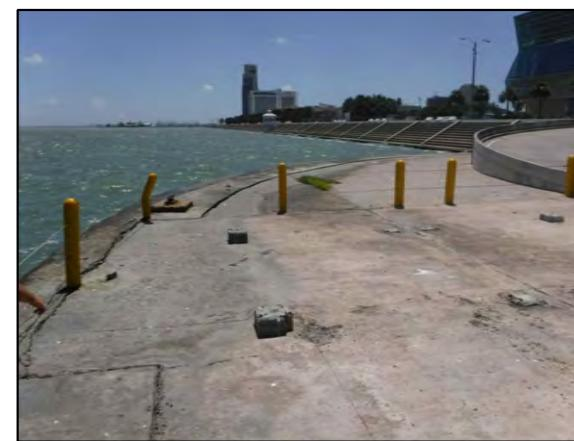
2 REMOVE AND REPLACE DAMAGED BOLLARDS
