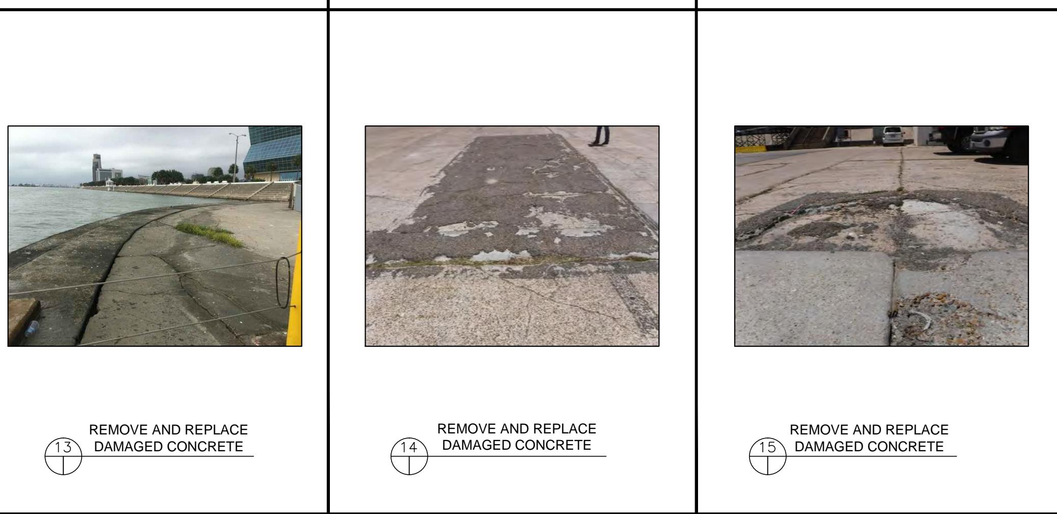
15 REMOVE AND REPLACE DAMAGED CONCRETE
