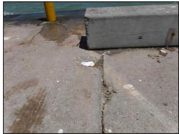
12 CLEAN AND REPAIR CONCRETE SPALLING
