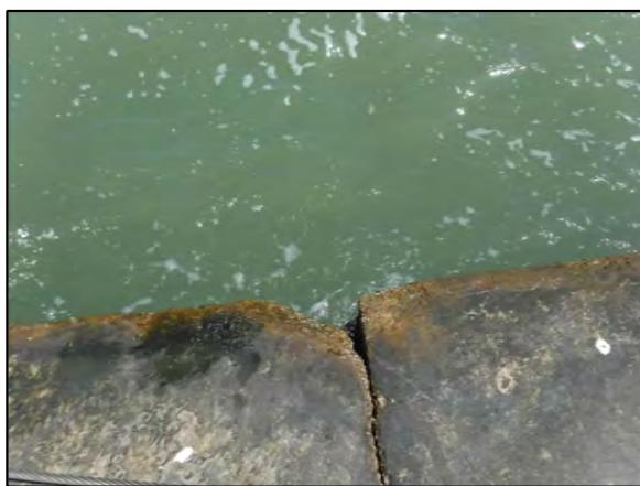
4 REPAIR DAMAGE TO CONCRETE BULKHEAD CAP
