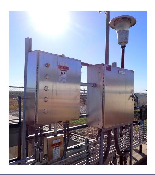
The spillway gate hoist control panels are exposed to the elements and extreme heat.
