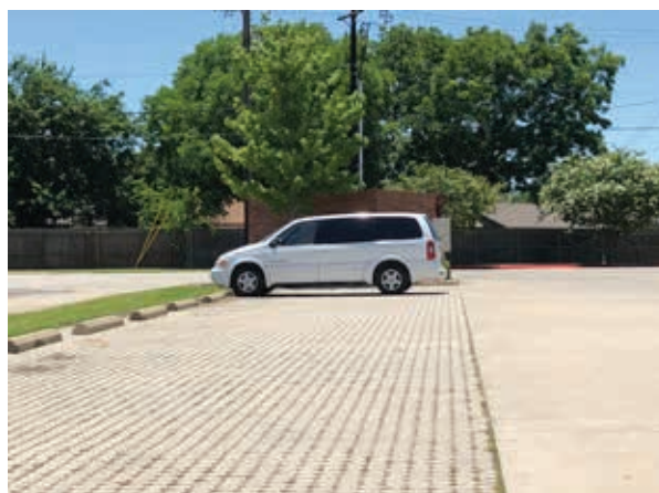
Example of Permeable Parking Surface
