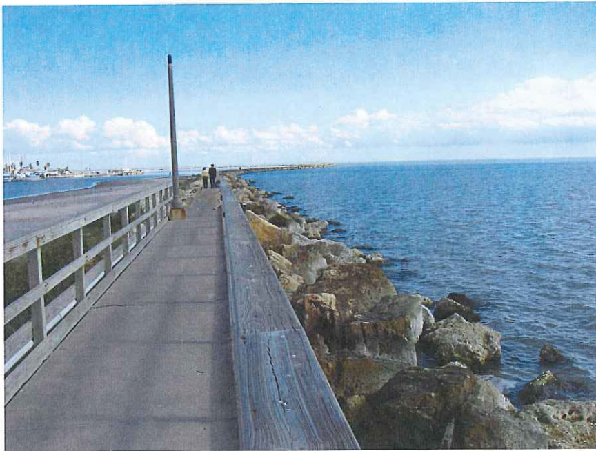
Figure VIII-3. Existing breakwater and walkway, facing north.
