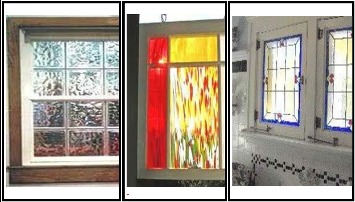
Figures 6.14.10.A.2.b. Block Glass & Stained Glass Windows
