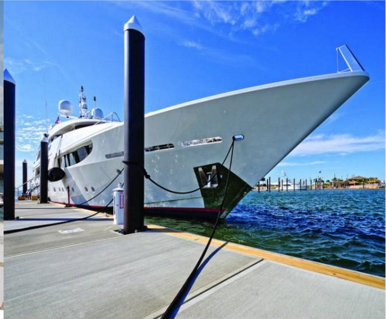
Pelican Rest Marina located in Galveston, TX, is Texas' newest megayacht marina featuring concrete floating docks by Bellingham Marine and catering to boats 60' and larger.
