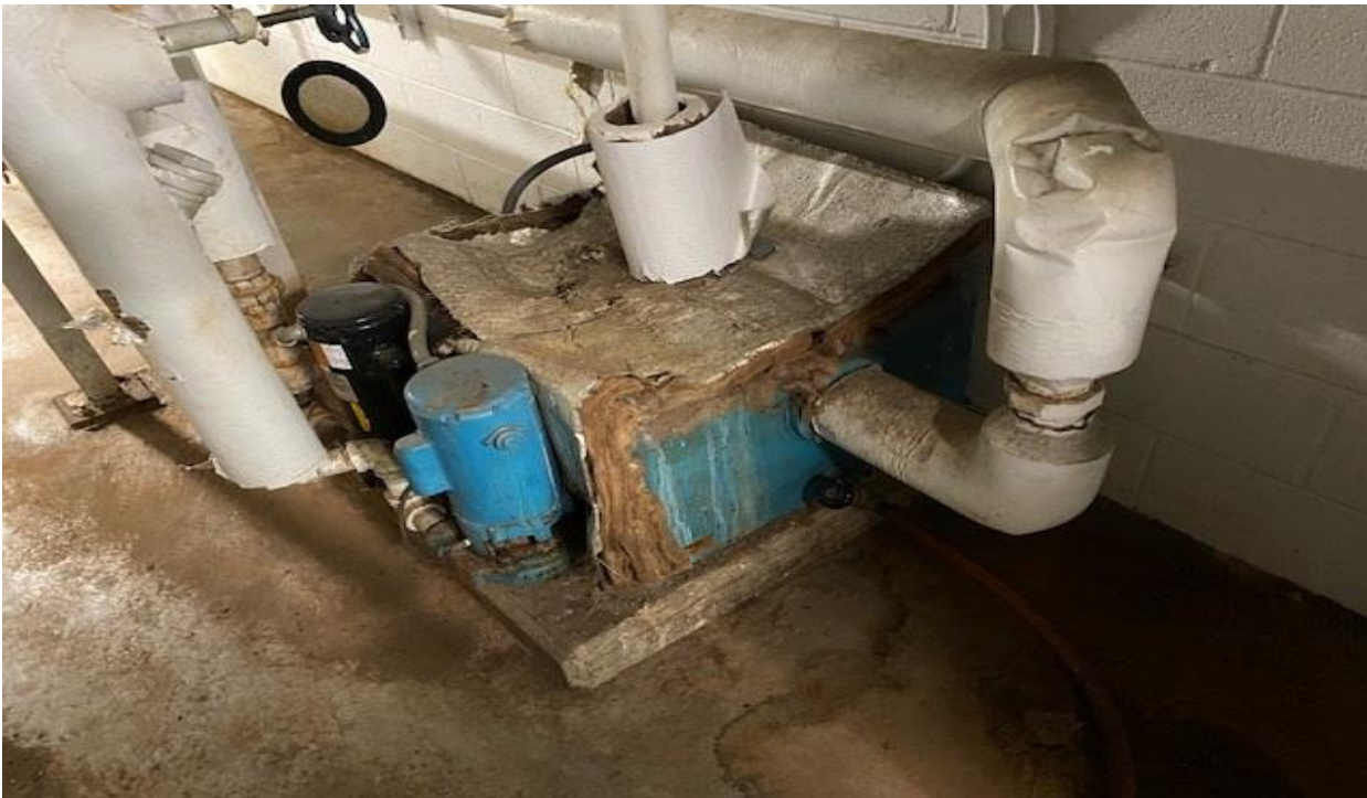
Condensate Return System #31 – Engine Cleaning Mechanical Room
