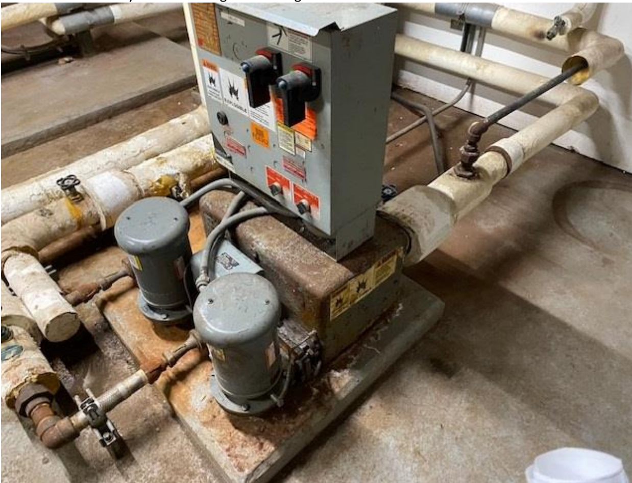
Condensate Return System #31 – Engine Cleaning Mechanical Room
