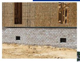
Requirements for Flood Openings in Foundation Walls and Walls of Enclosures
