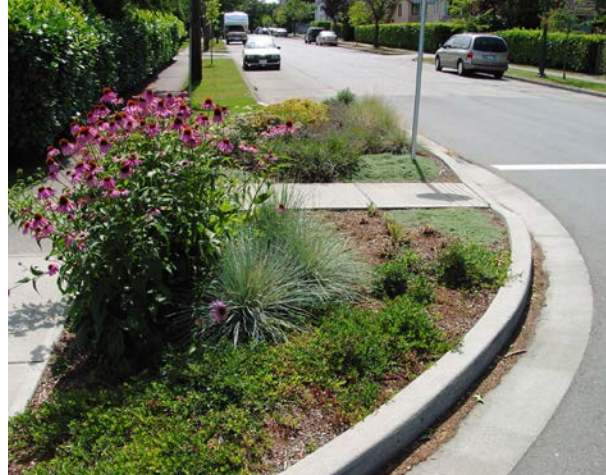
Curb extensions help to slow traffic by reducing lane widths at pedestrian crossings while offering beautification opportunities
