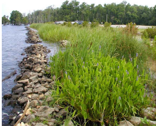
Living shorelines provide a more beautiful bayside environment while fostering greater resilience to coastal erosion
