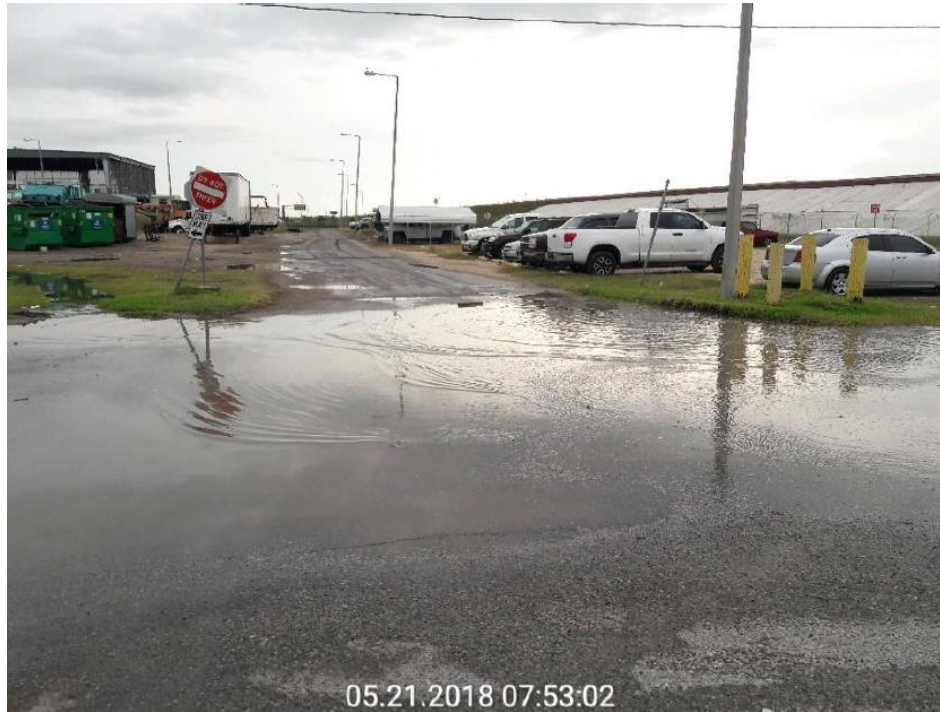
Citizen's Collection Center and Transfer Station Exit
