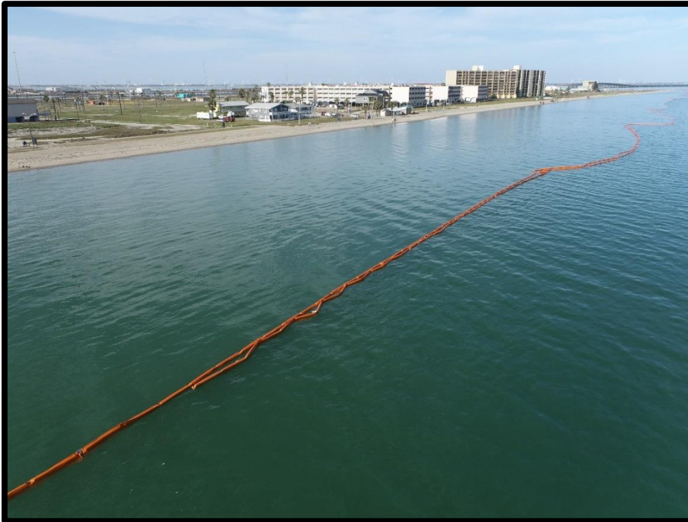
Photograph 5: Protective boom deployed along North Beach.
