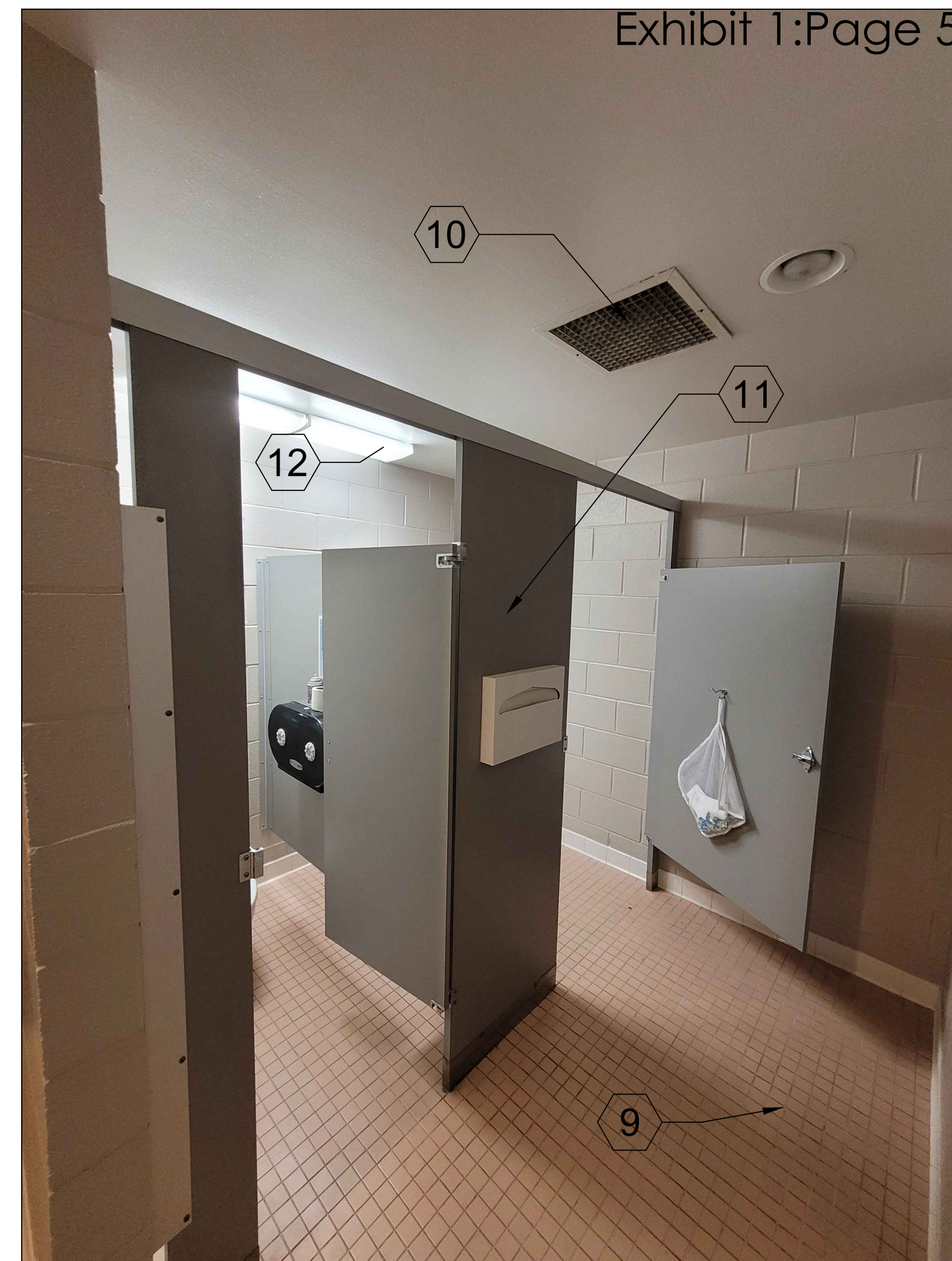
3 PHOTO - WOMEN'S TOILET STALLS X X N.T.S
