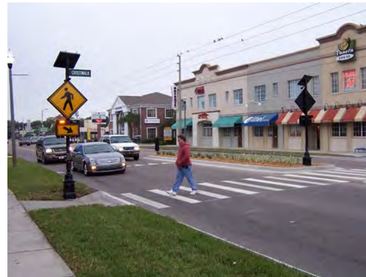
(Top left) Angled median break forces bicyclist to face the direction of traffic he is about to cross. (Top right) High visibility ladder markings and median island at bicycle boulevard crossing. (Bottom Left) Rectangular rapid flashing beacons (RRFBs) at midblock crossing. (Middle right) Signalized crossing for a sidepath connecting two bike boulevard segments. (Bottom right) Pedestrian hybrid beacon with colored pavement bicycle crossing.
