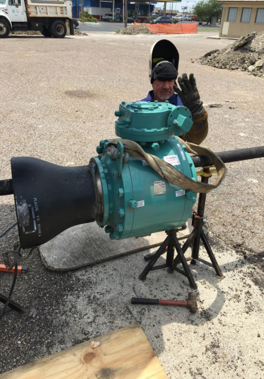
10" Ball Valve Installation- Gollihar Project
