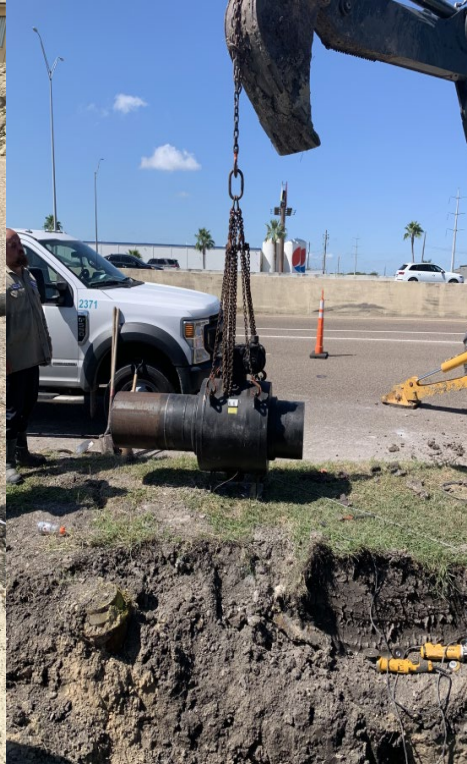
16" Ball Valve Installation- Columbia Project
