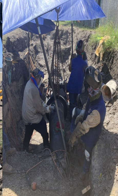
16" Ball Valve Installation- Columbia Project
