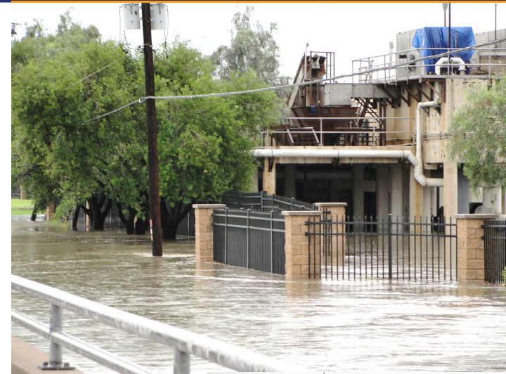
Greenwood Wastewater Treatment Plant
