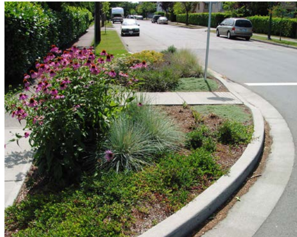
Curb extensions help to slow traffic by reducing lane widths at pedestrian crossings while offering beautification opportunities Photo Credit: Richard Drdul
