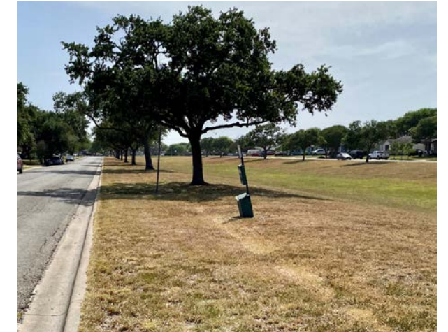
Brawner and other drainage greenways provide an opportunity for further investment into shared use paths to support existing uses.
