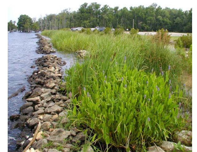
Living shorelines provide a more beautiful bayside environment while fostering greater resilience to coastal erosion Photo Credit: nrcsolutions.org
