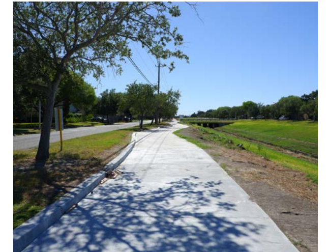
Schanen Hike/Bike Trail Along a Drainage Channel
