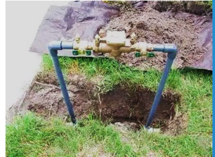
Reduced Pressure Assembly (RPZ) installed at the meter
