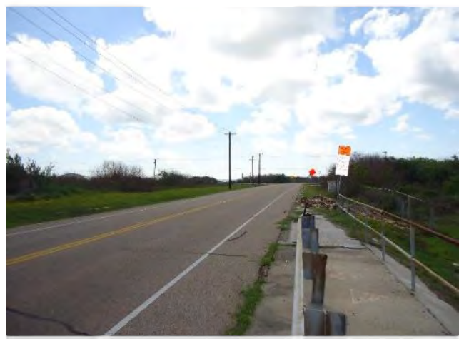
12. Hustlin Hornet Drive, viewing southeast, subject on right
