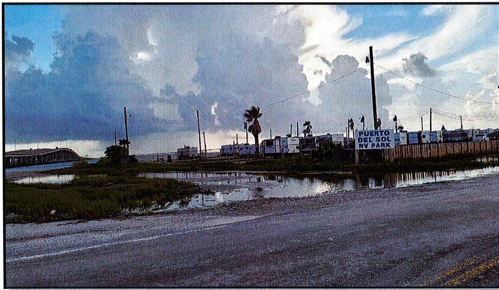
View looking northeast toward subject from Hull Street
