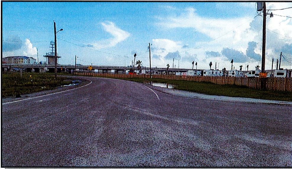
View looking northwest along Timon Blvd. Subject on right
