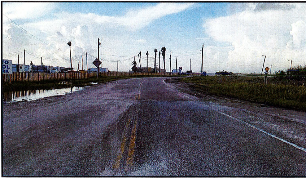
View looking east along Timon Blvd. Subject on left
