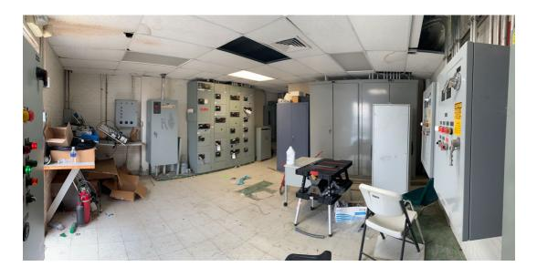
This area is being used for instrumentation work, PLC panel troubleshooting, and PLC panel assembly. This space was not designed to be an electrical workspace.
