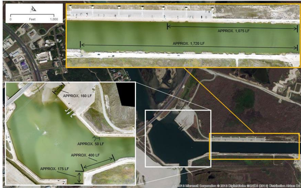
Figure 4 - Damage Locations within Reach 3
