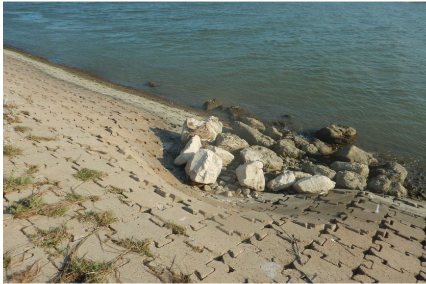
Figure 8 - Previous Repairs Using Riprap
