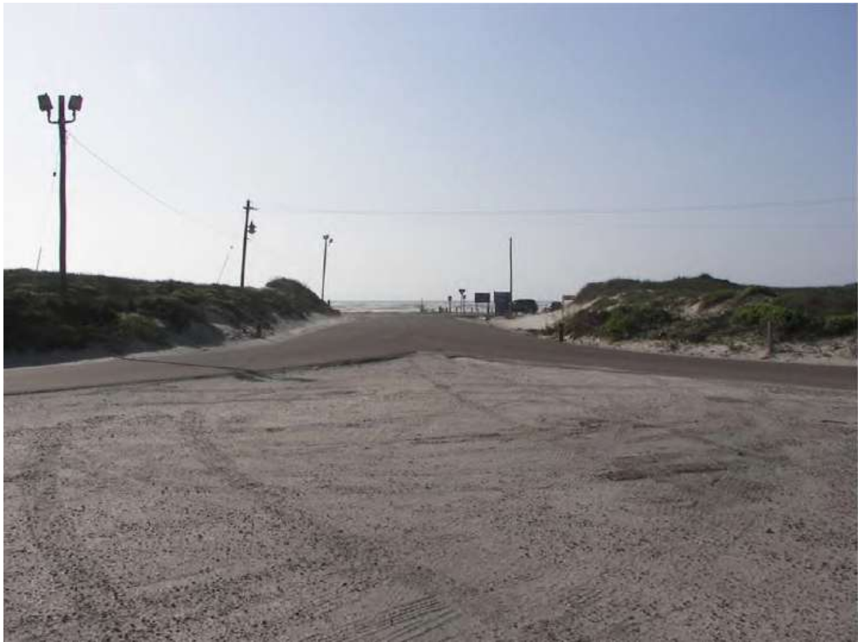
Figure 28: Padre Balli Park Entrance/Existing Road, Seaward View
