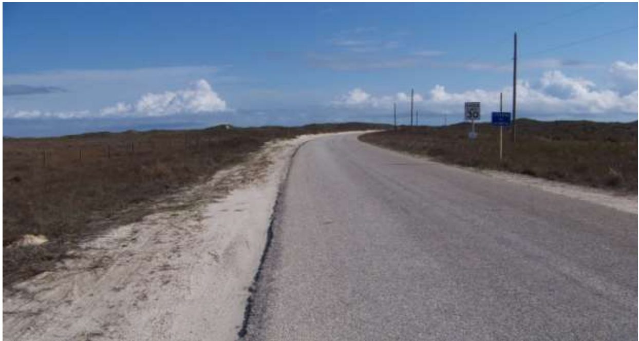
Figure 14: Beach Access Road 2, Seaward View Near State Highway 361
