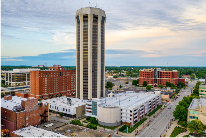
Wyndham 400 Rooms 30 Stories Springfield, IL
