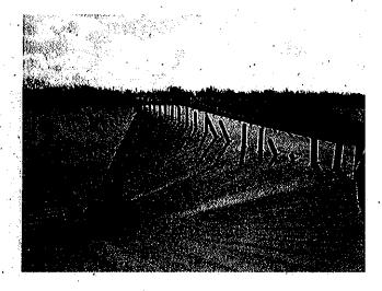
HDR Engineering, inc. Texas Registered Engineering Firm F-754 555 N. Carancahua Sulto 1690 Corpuș Christi, TX 78410-0850 Phone: (361) 696-3300 Fax: (361) 696-3385 www.hdrinc.com 2. The west bank of the outfall channel, north of FM 70, where two pipelines have been undermined by erosion -
