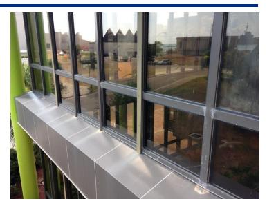
Replacement of the existing two story aluminum and glass curtain wall system and upgrades for wind-storm certification.
