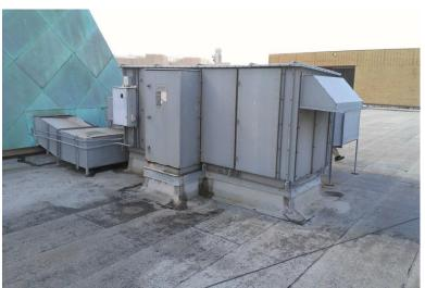
Alt. #2: Replacement of the roof-mounted air-handler unit installed with the original building construction.
