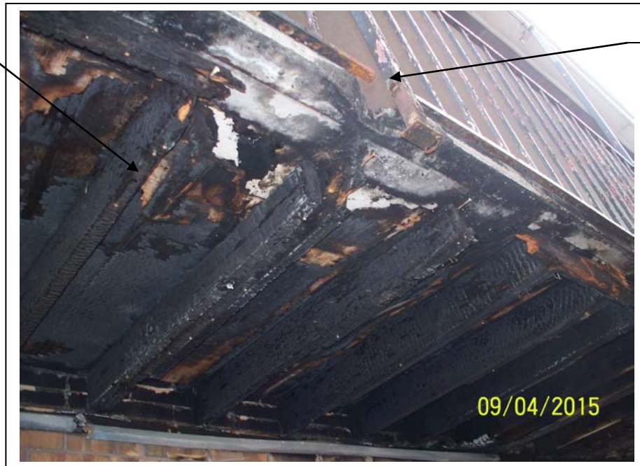
Photograph No. 8 – Fire Damage at Exterior Walkway
