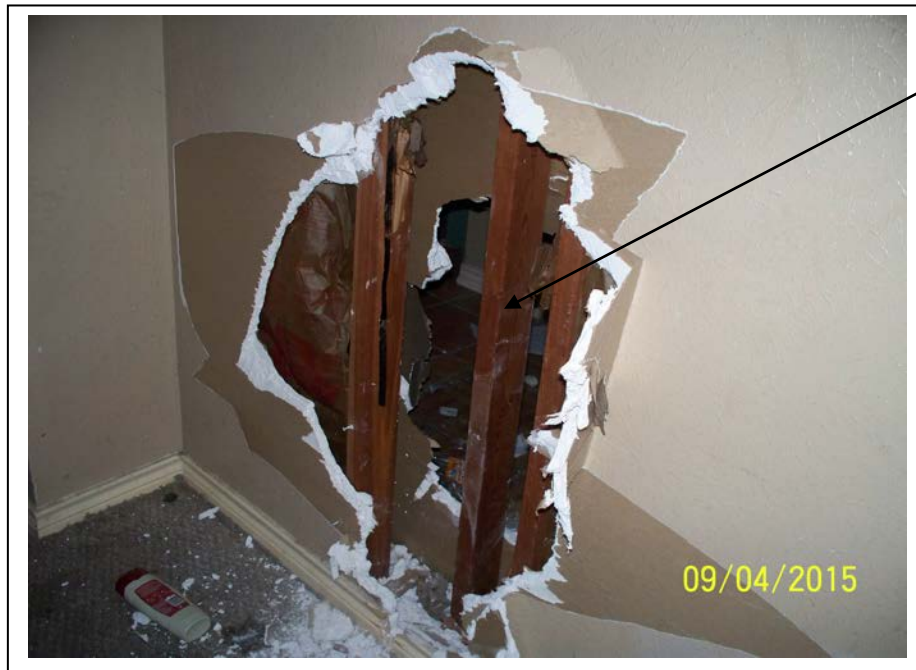
Photograph No. 10 – Typical Interior Framing
