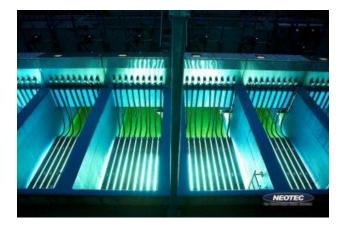
Provides new UV system to meet current TCEQ permit limits. The existing system is at end of its useful life and was not designed to address Enterococci Bacteria.
