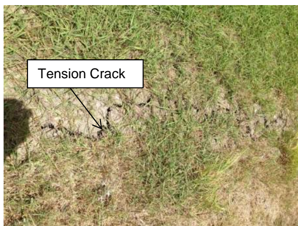
Figure 8 – Tension Crack (July, 2016)
