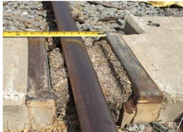
Figure 31- Asphalt Infill Material
