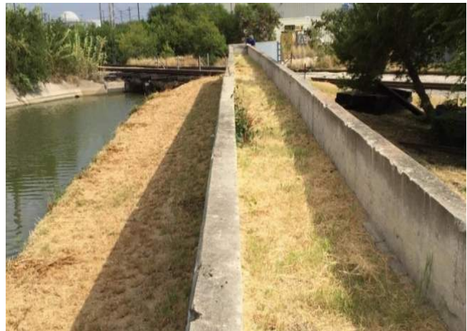
Figure 22 – Top of Wall (missing concrete)
