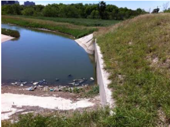
Figure 10 – Concrete Headwall and Basin
