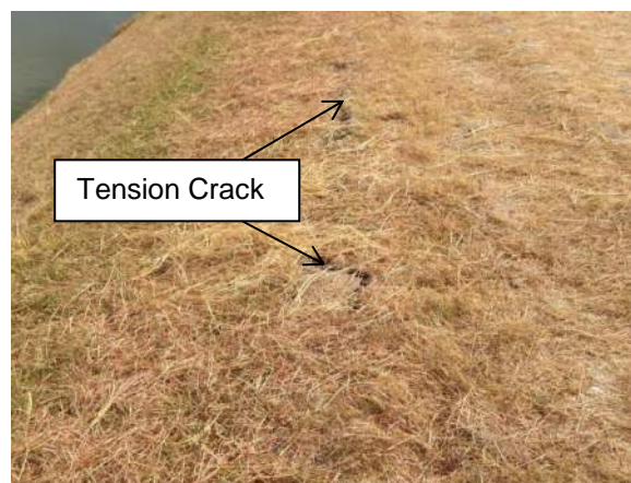
Figure 9 – Tension Crack (August, 2016)
