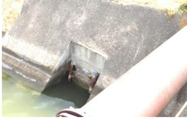
Figure 33 – Typical Flap Gate
