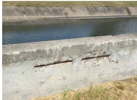
Figure 24 – Exposed Rebar (Front of Wall)
