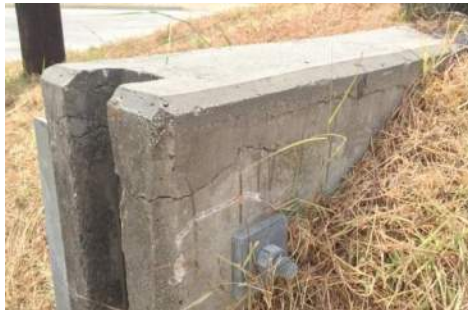
Figure 29 – Delaminated Concrete Support
