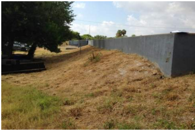
Figure 23 – Backslope of Crib Wall
