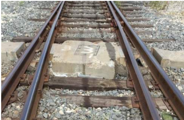
Figure 30 – Gaps Adjacent to Railroad Tracks
