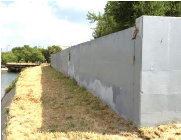
Figure 21 – Front Face (spalls/exposed rebar)
