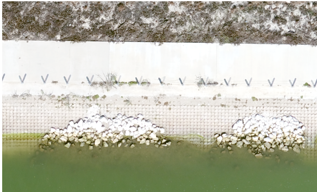
Figure 10 – Example of previous repairs constructed by capping damaged ABM in-place with riprap.
