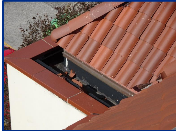
Water Infiltration Area
