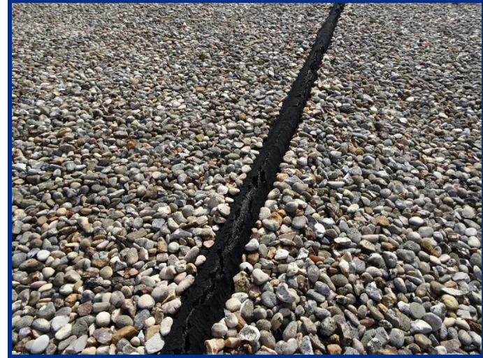
Deteriorated Roof Joint
