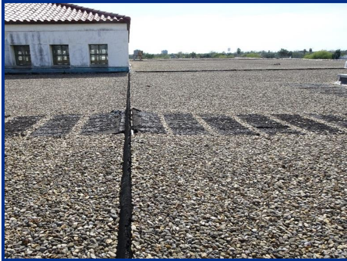
Deteriorated Roof Joint
